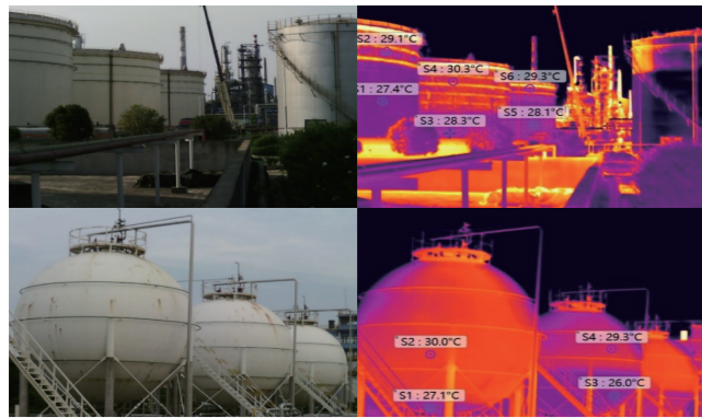
储油罐液面、沉淀检测
